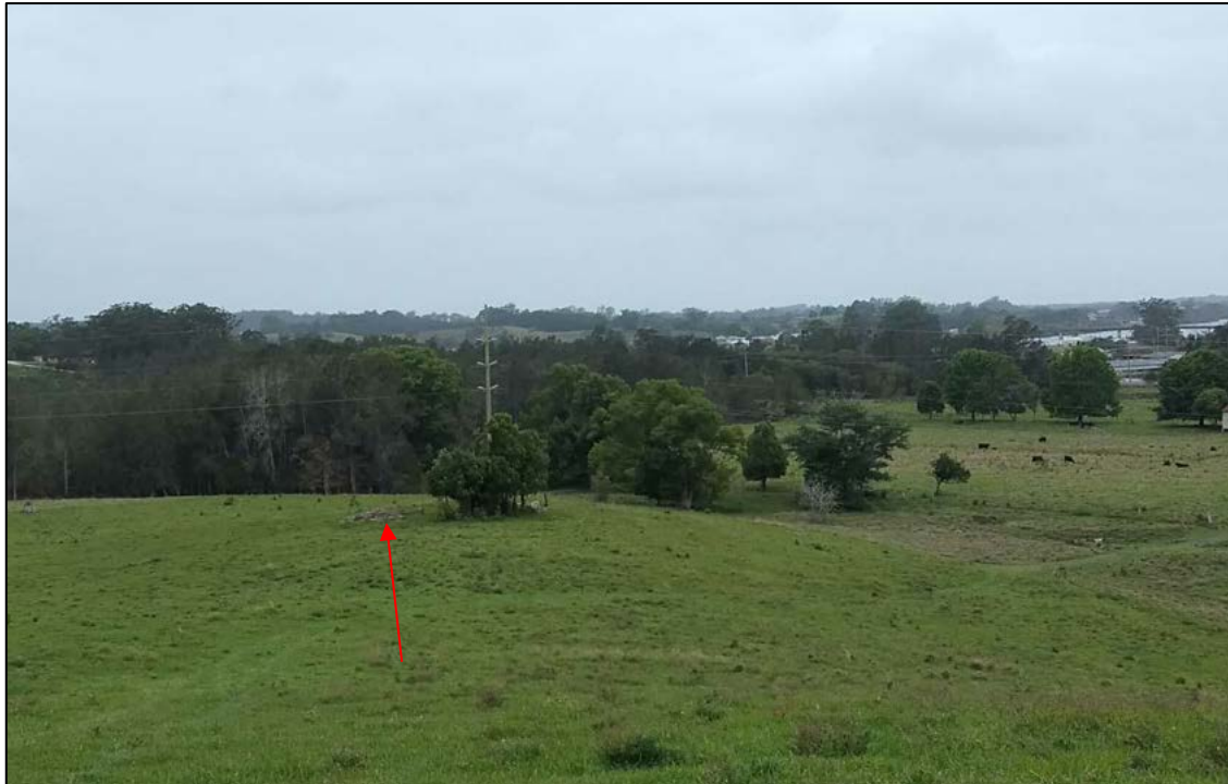
Photograph 13: High voltage power lines with discarded timber, located in central portion of the site, facing east (17 November 2020).
